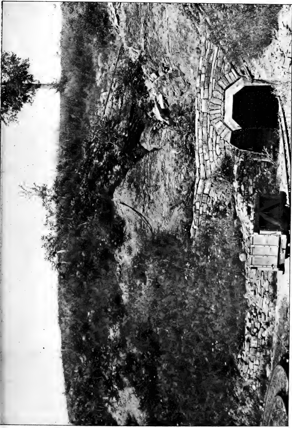
Entry to the mines of the Franklin Iron Manufacturing Co., Clinton. Red flux bed appears near top, its lower portion being indicated by the iron pipe.
